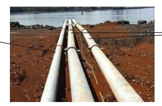
Sphere Lock<sup>™</sup> couplings allow for angled/offset connections.
